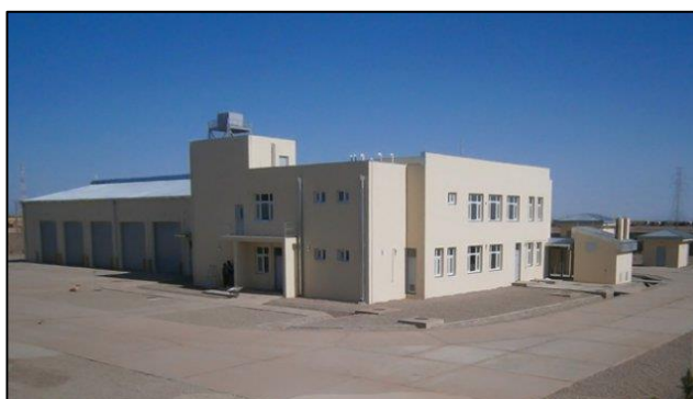
Figure 2. Fire Station Built for Afghan National Police
